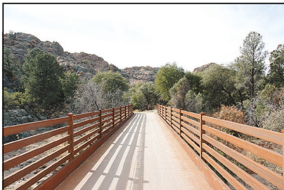
All bridge decks are actual flatbed rail cars.
