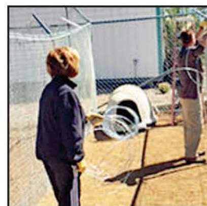
Dave and Veronica installing wire
