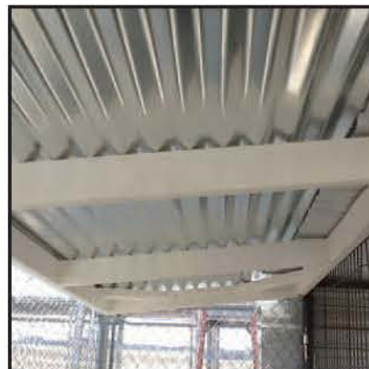
New roof inside
