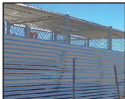
After - long wall exterior
