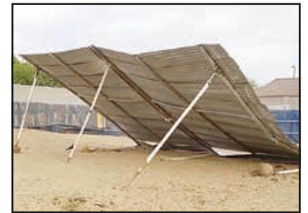
Destroyed shade cover
